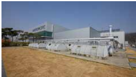
Expansion of the rainwater storage facilities
