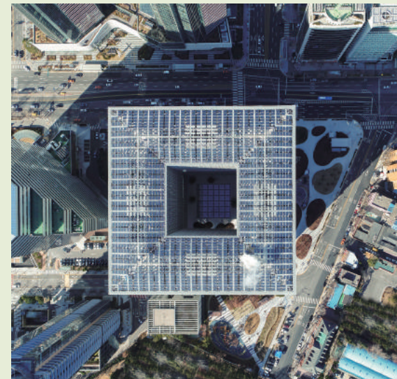
Photovoltaic Panel on the Rooftop of the New Headquarters
